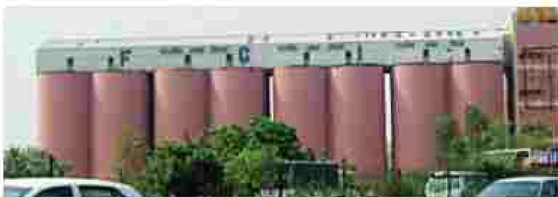
Fig. 1.10 (a) : Silos for storage of grains
